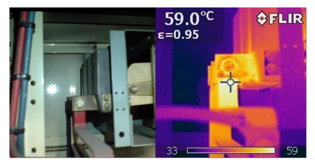
The Red phase supply of P36 MCC Isolator situated inside the Plant shows evidence of heat, the load is equal between phases. The Rph - 59°C, in relation to the other 2 phases. Need to be repaired as time permits, Class 2.
